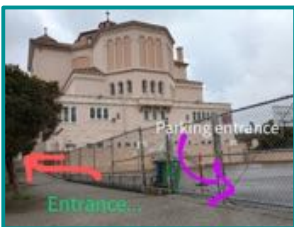
Our entrance below the rose window on Funston St.
